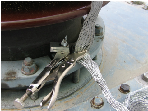
Fig. 4: Clamping aluminium braid for ground contact
